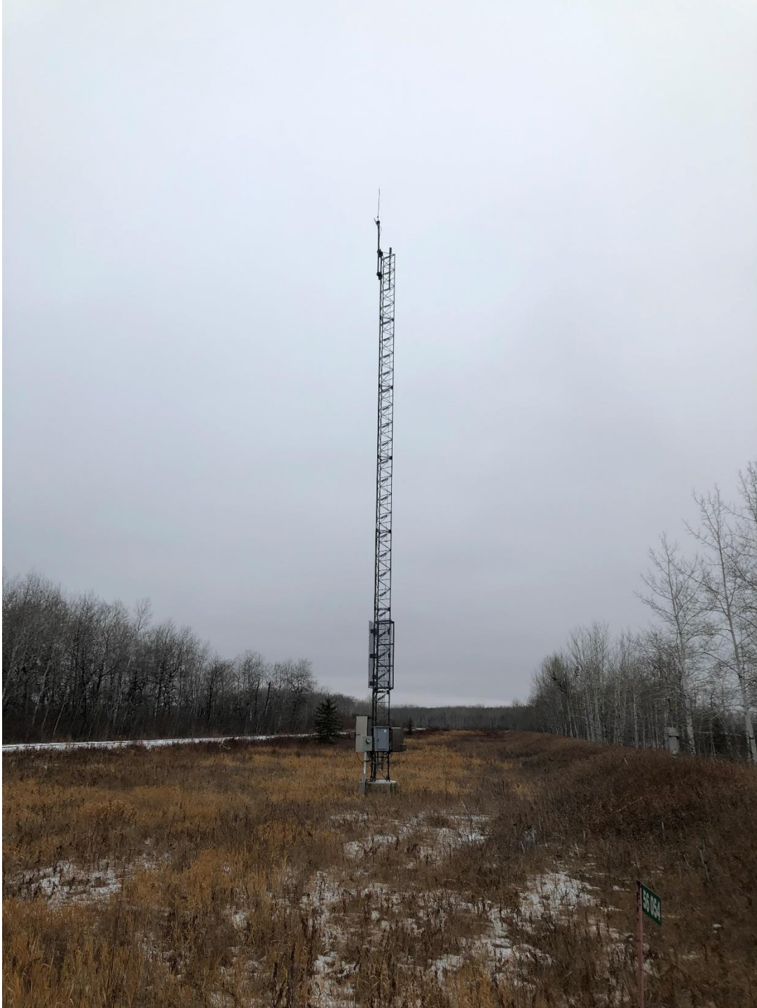
Figure 1: Mile 29.76 Communication Tower
