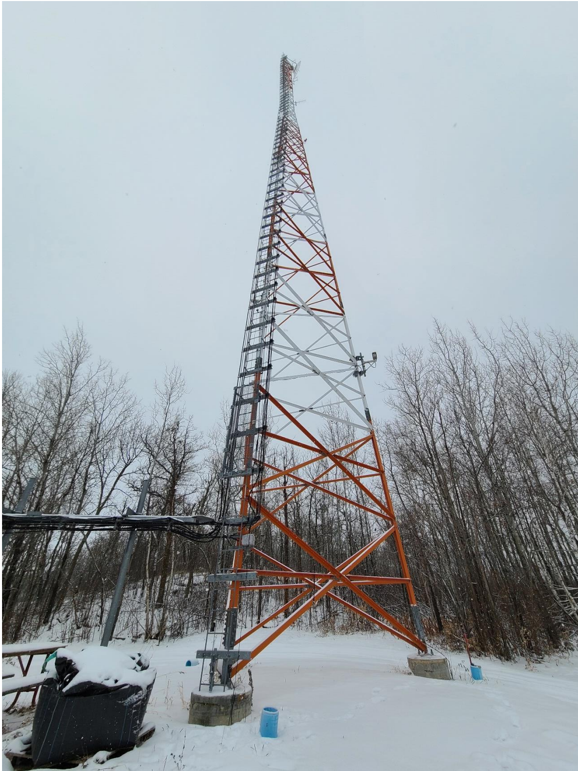
Figure 1: Shoal Lake Intake Communication Tower
