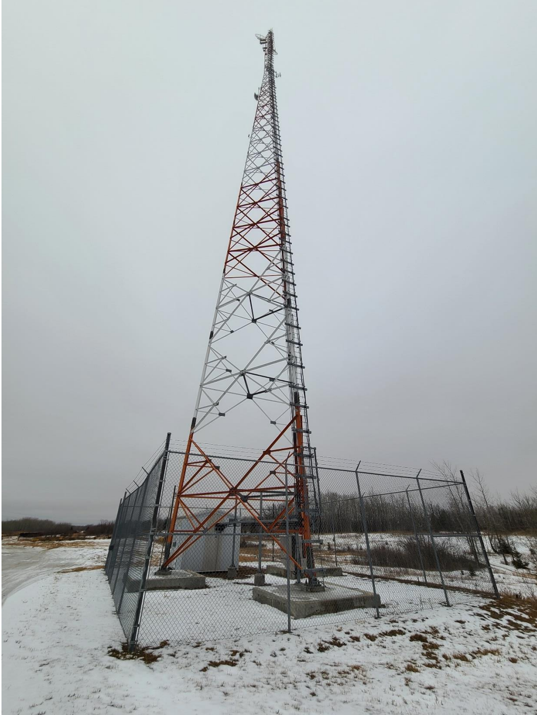
Figure 1: Ross Yard Communication Tower
